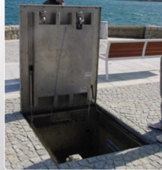
Liffey Service Tunnel - Dublin
